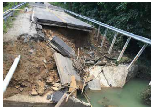
Image 15: Route 4 near Kanawha and Clay County lines washed away during flooding
