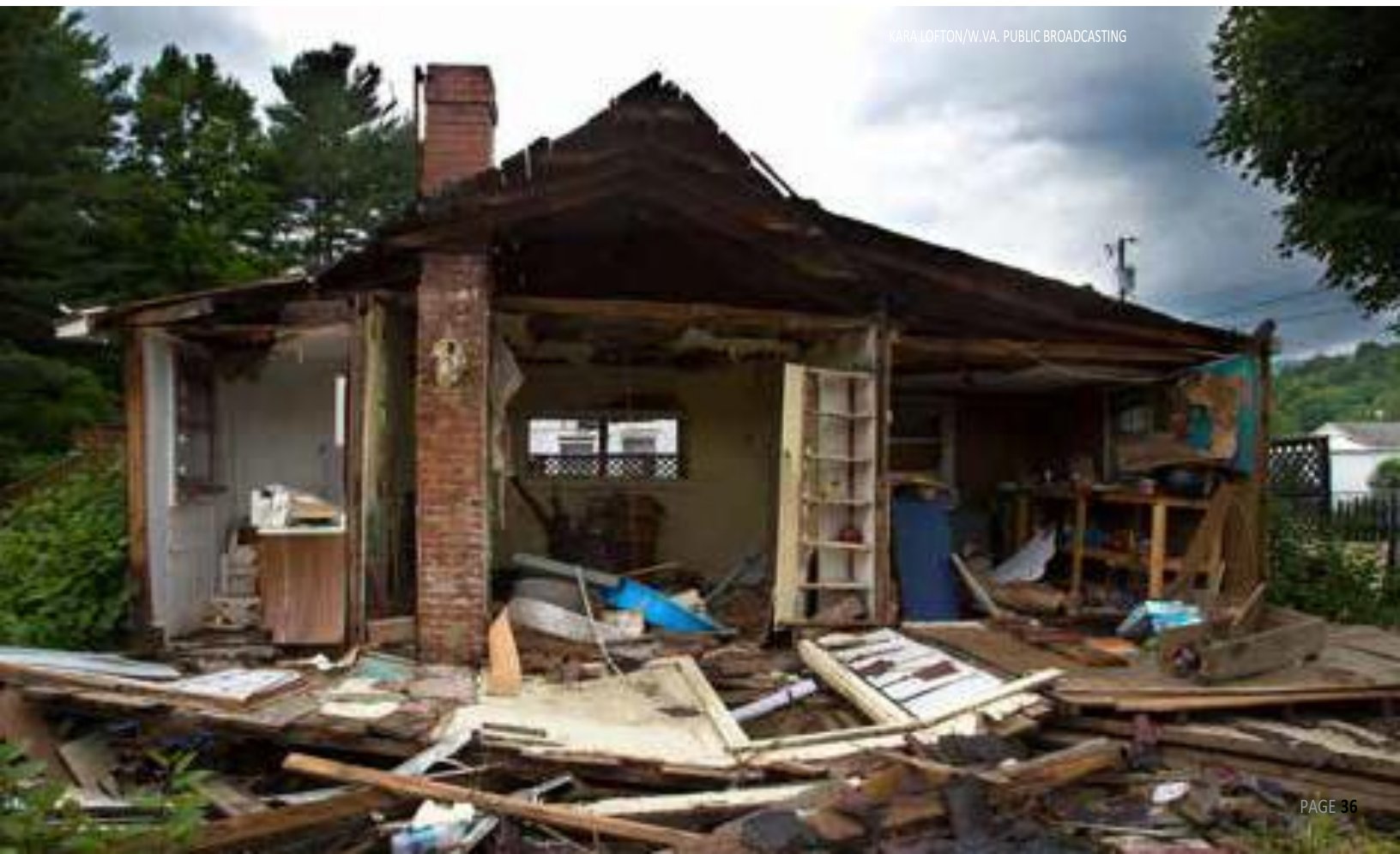
Image 10: A home destroyed by flood damage.
