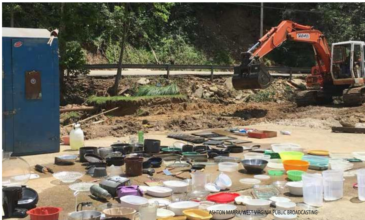
Image 1: An excavator rebuilds where a private bridge once stood while containers from a flooded kitchen are laid out to dry
