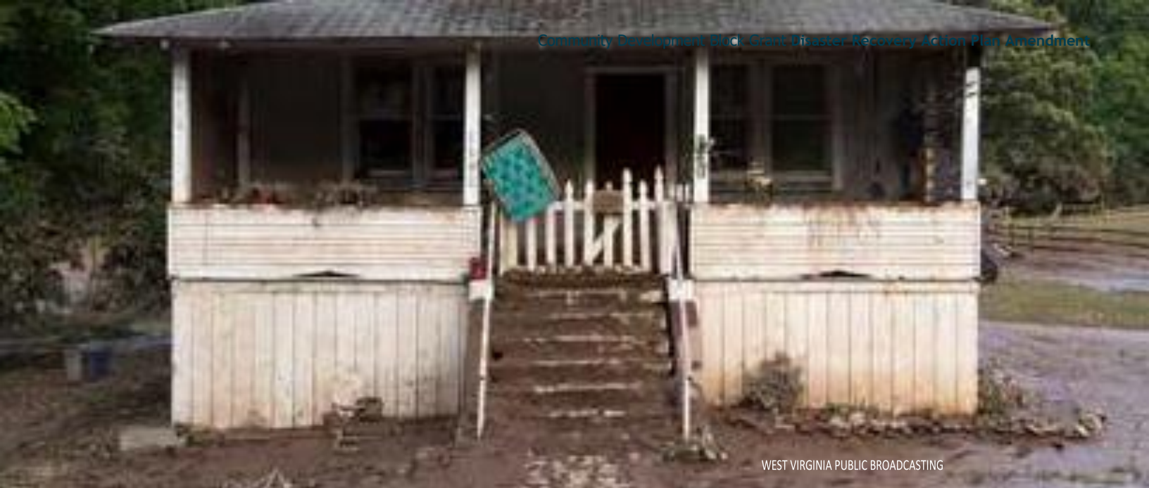
Image 18: Damaged home in Clendenin
