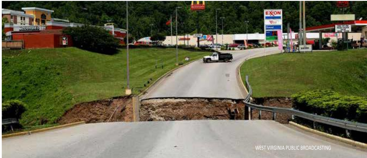
Image 20: Collapsed bridge at the Crossing Mall in Elkview
