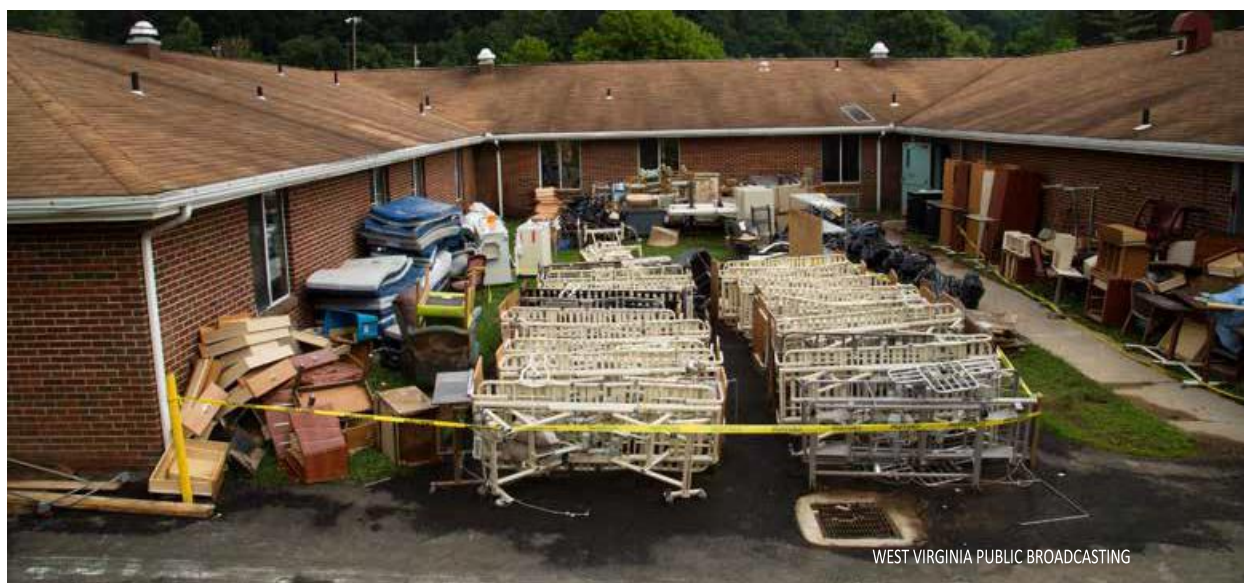
Image 14: The back of Nicholas County Nursing Home several days after the flood
