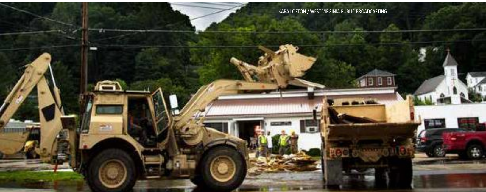
Image 23: Cleaning up flood damage in Richwood.
