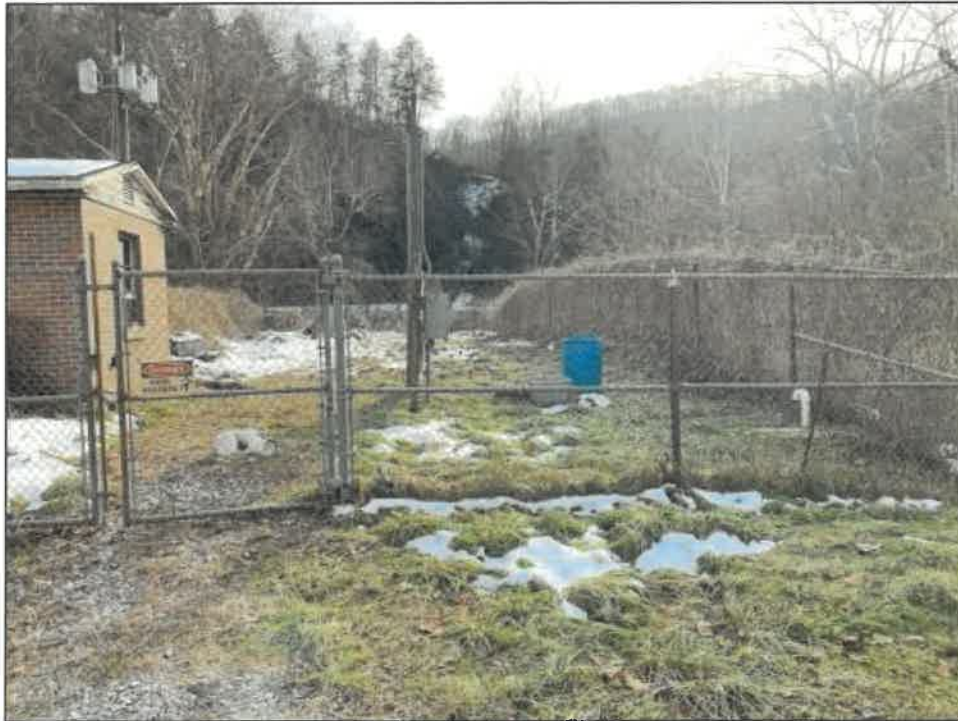
Pump Station No. 1 -- also known as "Two Run Station" (Lat: 38' 28'31", Long: -81 4'53")
