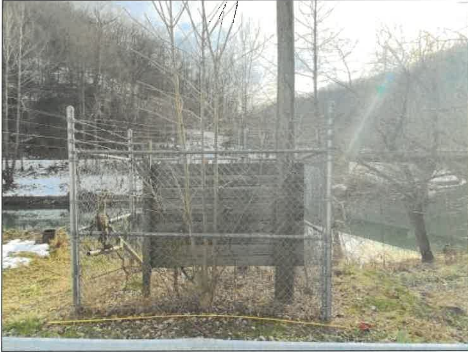
Pump Station No. 3 (no other name designated) (Lat: 38 27'38", Long: -81 5'16.5")
