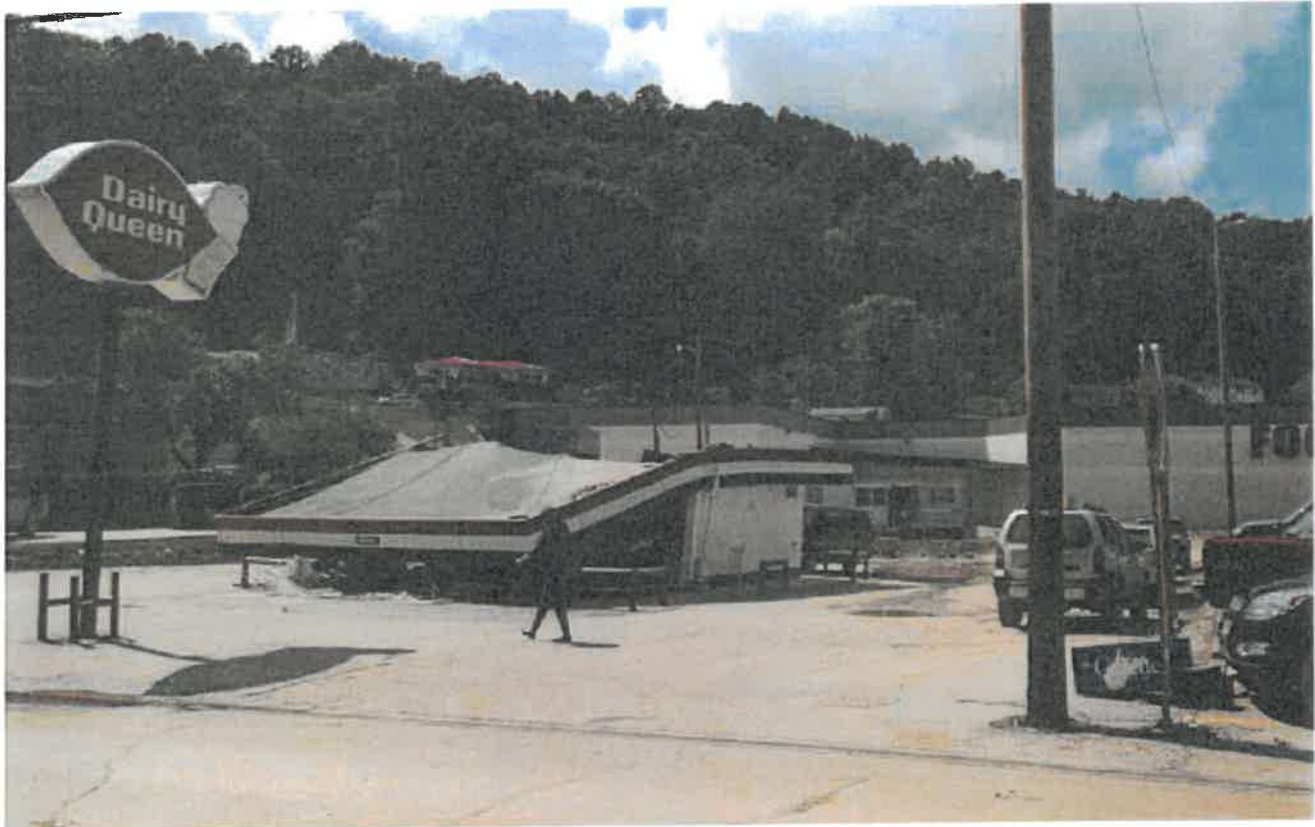
Image 8: A collapsed Dairy Queen as a result of flood damage
