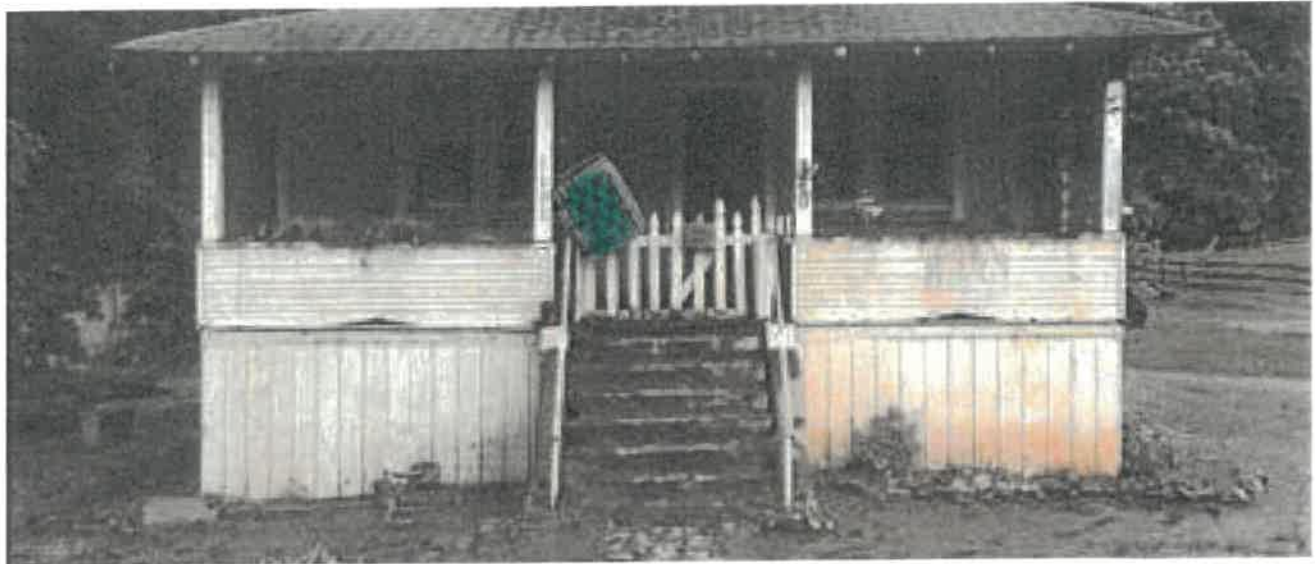
Image 18: Damaged home in Clendenin
