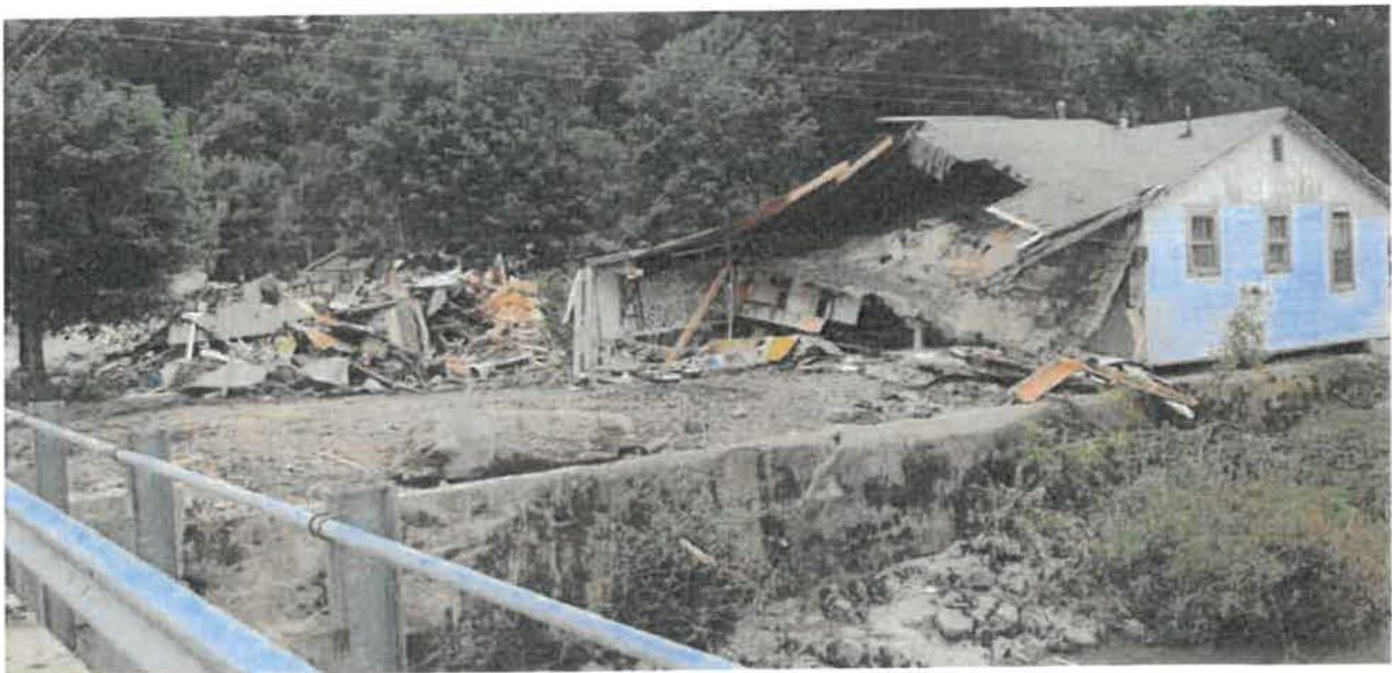
Image 21: Home destroyed by flood waters.
