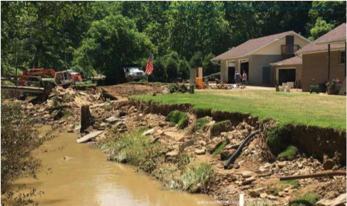
Image 25: An excavator, left, attempts to rebuild the piece of land where a private bridge used to sit. The bridge was washed away by flood waters.
