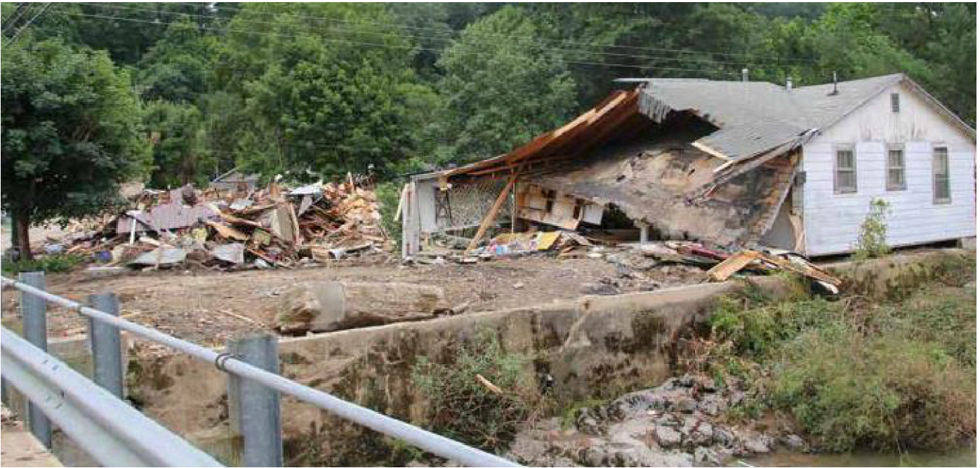
Image 21: Home destroyed by flood waters.
