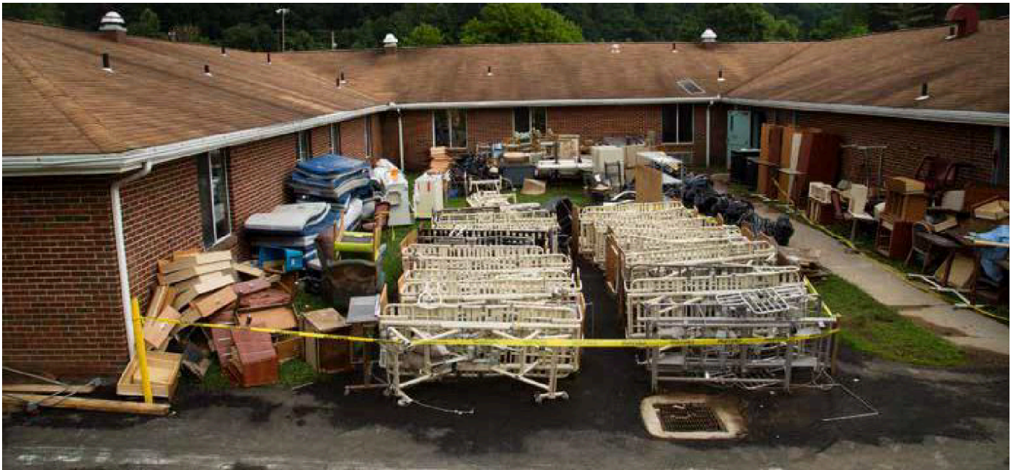
Image 14: The back of Nicholas County Nursing Home several days after the flood
