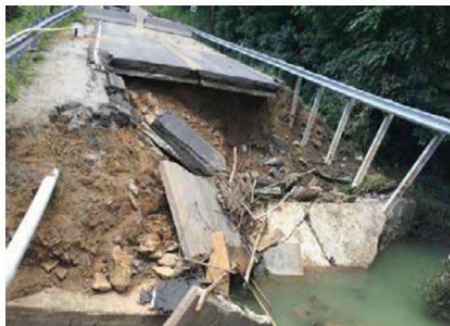
Image 15: Route 4 near Kanawha and Clay County lines washed away during flooding
